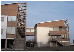
Chesapeake Bay Foundation, Annapolis, Maryland, 2000, Smith Group
