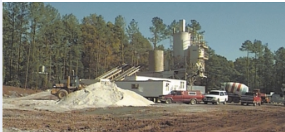
On-site concrete batch plant
